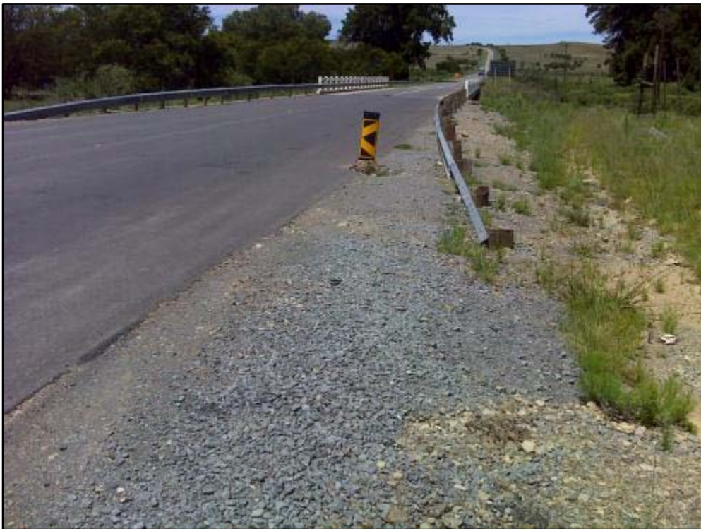
Figure 4. Example of associated road infrastructure (bridges).
