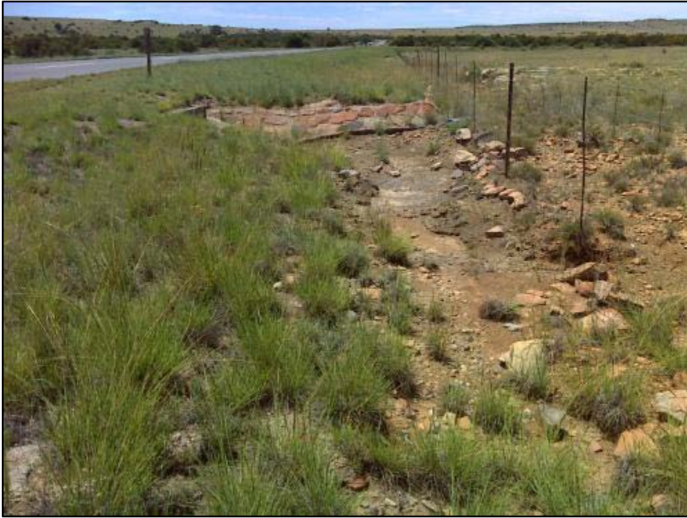
Figure 3. Example of road associated road infrastructure (water channels).
