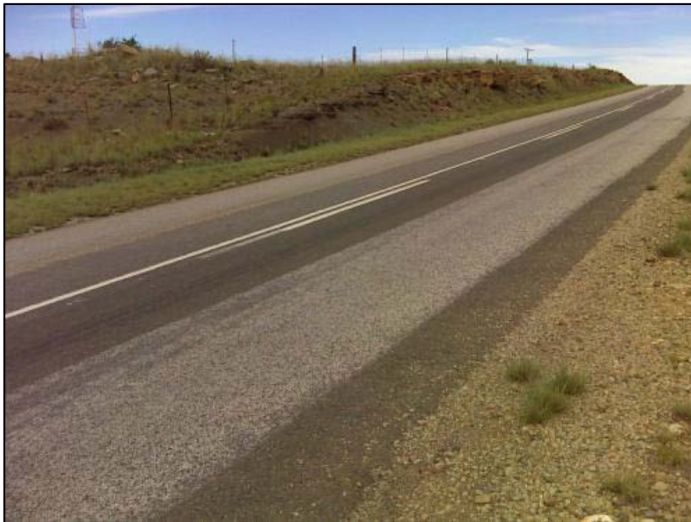
Figure 2. Example of a rocky outcrop extending beyond the road reserve.
