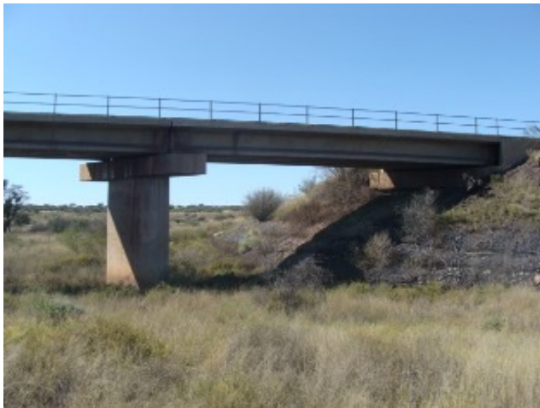
Figure 7: Closer view of existing bridge.
