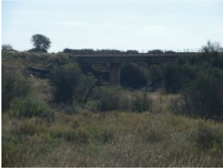
Figure 6: Existing rail bridge over the Gamagara River.
