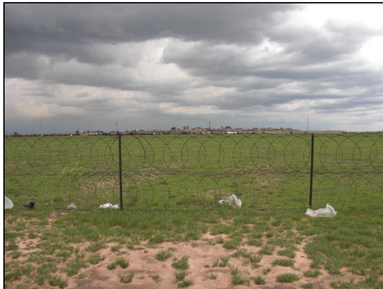
Figure 12: General view of the waste site and fenced buffer zone
