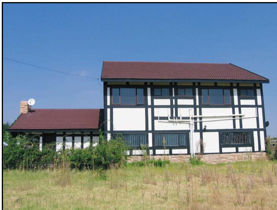
•Figure 2. Building photographed from the north
