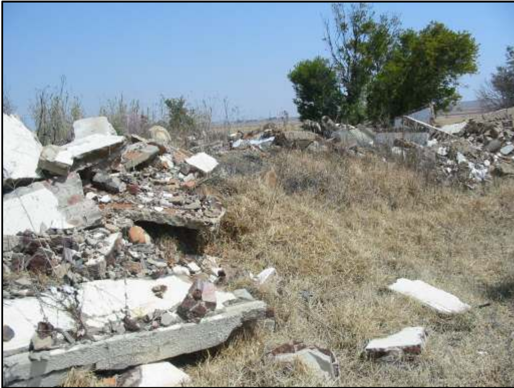
Figure 1: Demolished remains of house
