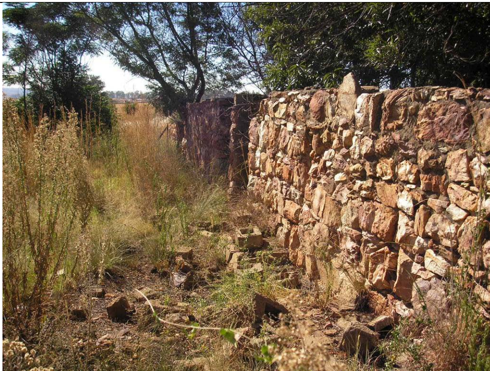
Fig. 4. The front side of the structure.
