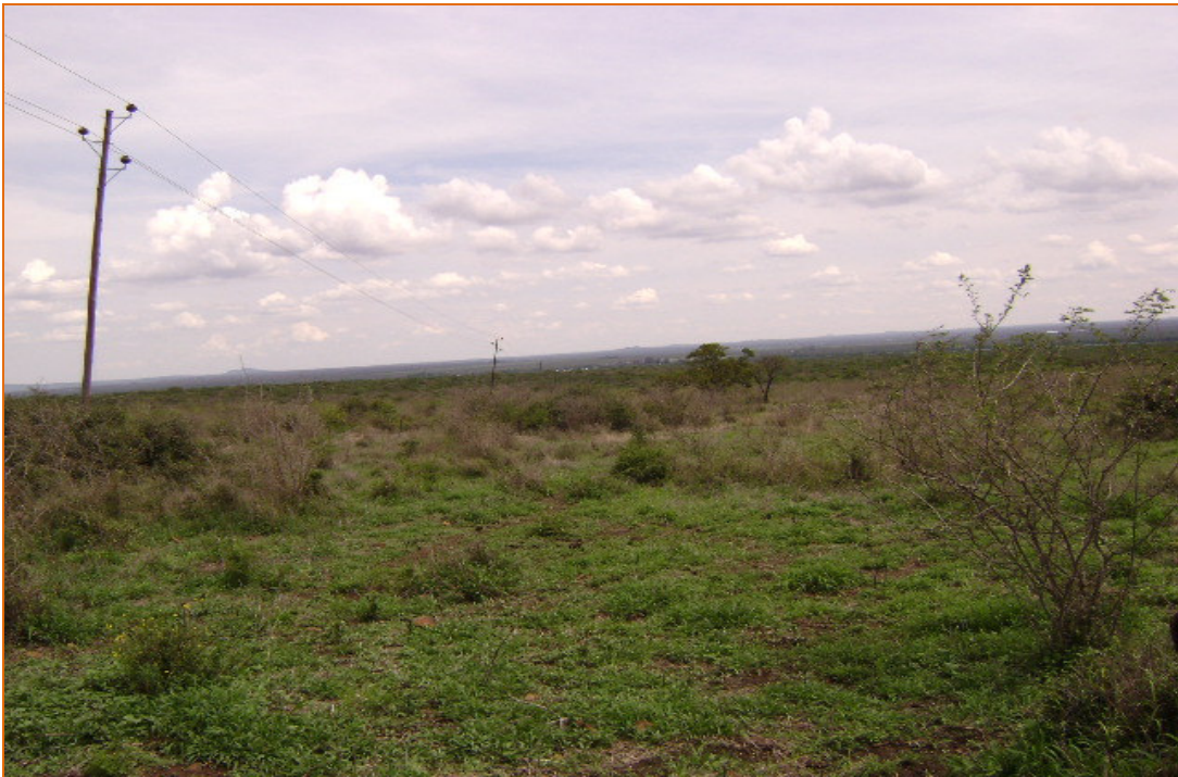
Figure 2: View of the existing electricity power line across the proposed site.
