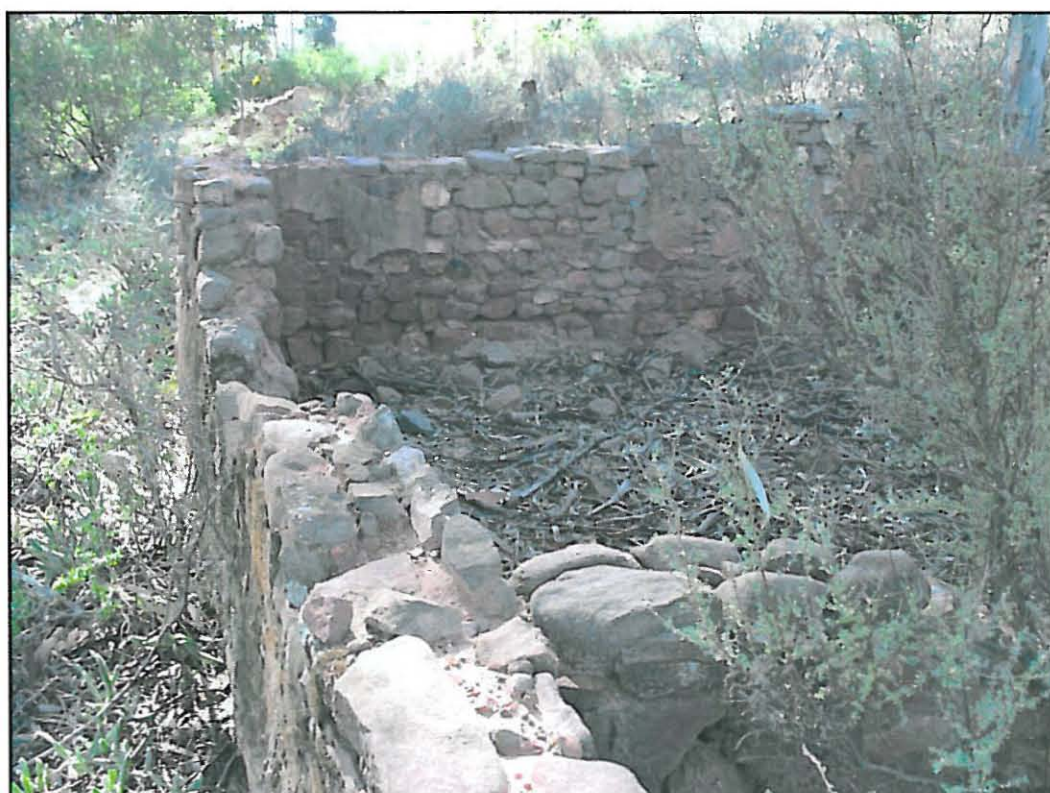
Figure 20: Close-up of the walls of the central structure showing the traditional construction methods employed at this site (MR531/2). The remains of the northernmost structure are just visible in the background.
