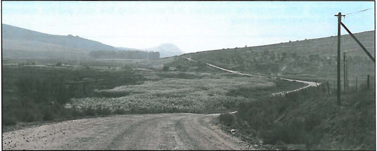
Figure 3: View towards the northwest from near the south-eastern part of the section to be upgraded.
