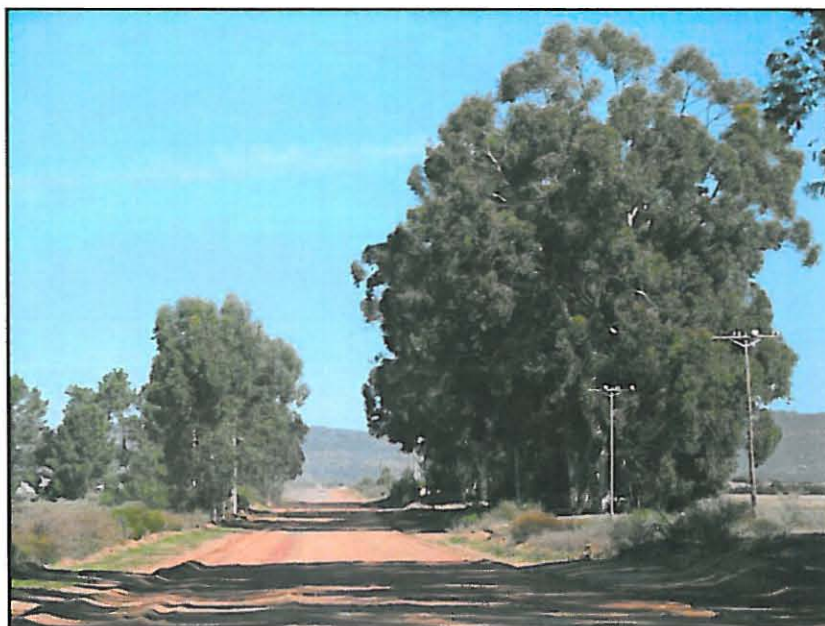
Figure 24: The tree line which falls partly within the road reserve (MR534/4).
