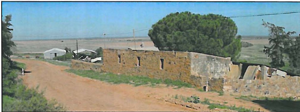
Figure 23: One of the structures located immediately alongside the MR534 and next to the Maclear Beacon site (MR534/3). The Beacon lies just beyond the left end of the stone building.
