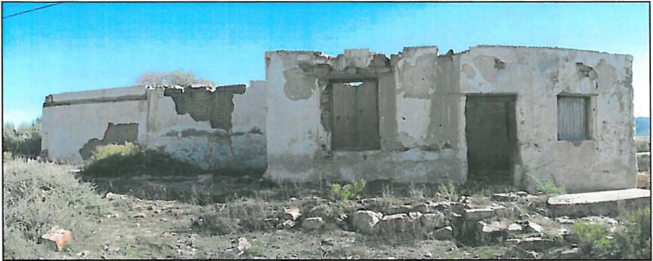
Figure 15: The rear (northern) side of the ruined house (MR531/4).
