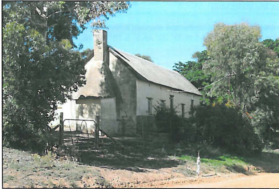
Figure 24: The house immediately across the MR534 from the Maclear Beacon site (MR534/3).
