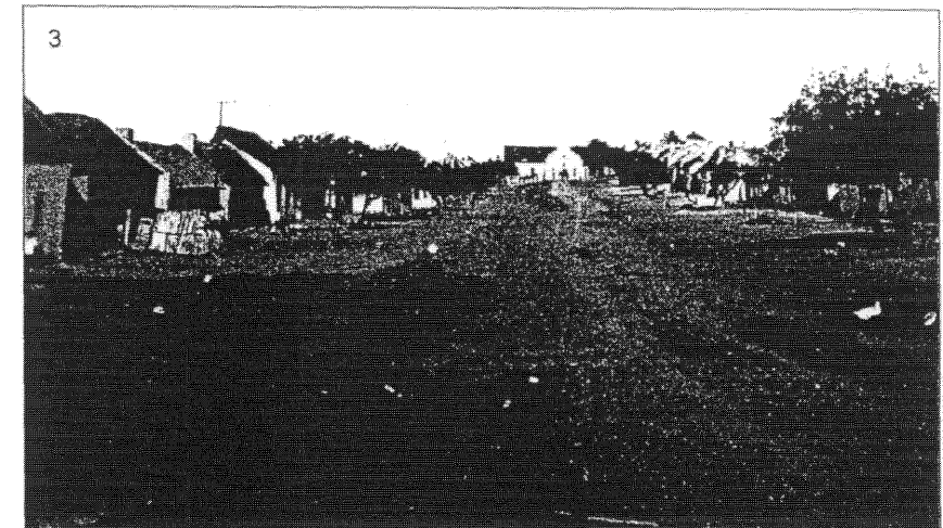
Plates 2 and 3 show Church Street, Elim as it is today and as it was at the end of the 19 th century. Levelling of the road has resulted in an undesirable cut which has very much altered the streetscape and character off the village. The Church is and always was the focal point of the village. Gutters and channels were informal.
