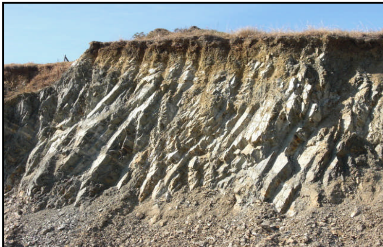
Figure 21: Close-up of the anthropic sterile section at the quarry site
