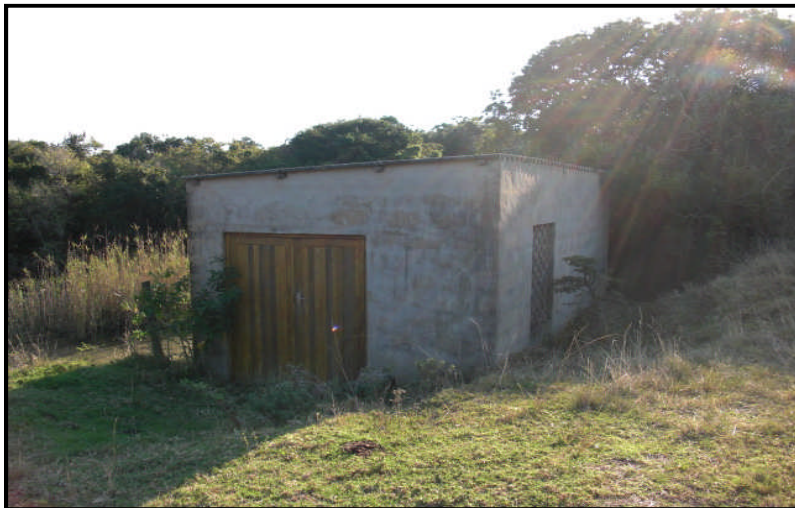
Figure 37: The C3 contemporary pump station
