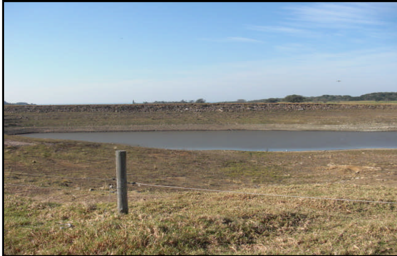
Figure 14: Close-up of the manmade dam
