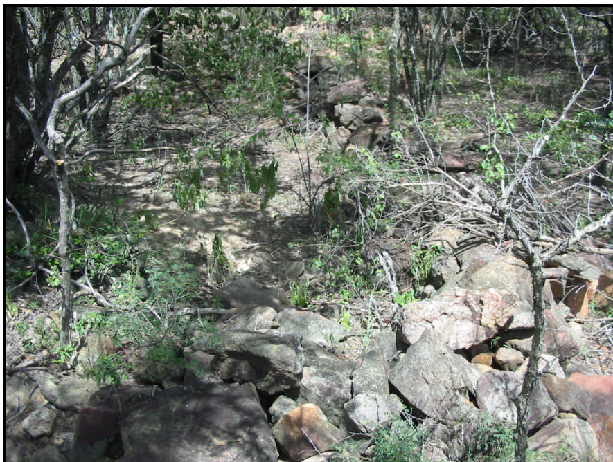
• Figure 4 : Overgrown stone walling
