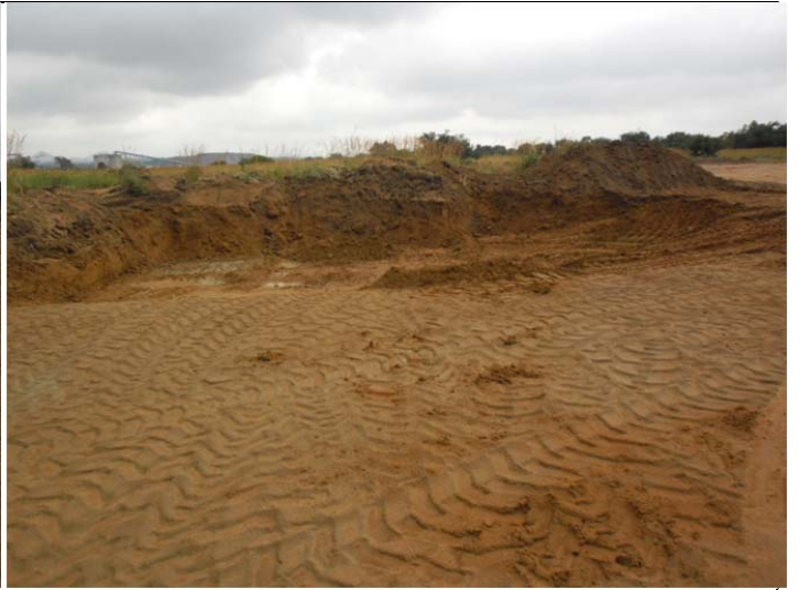
Figure 18. General Site conditions in the southern portion of the study area.
