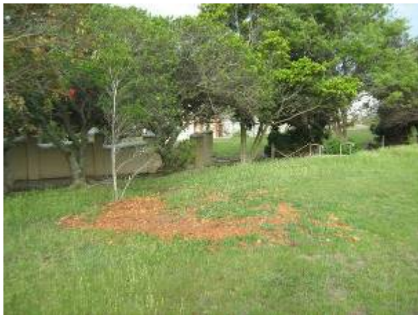
Fig. 11. One of the trial pits dug within the area proposed for development.
