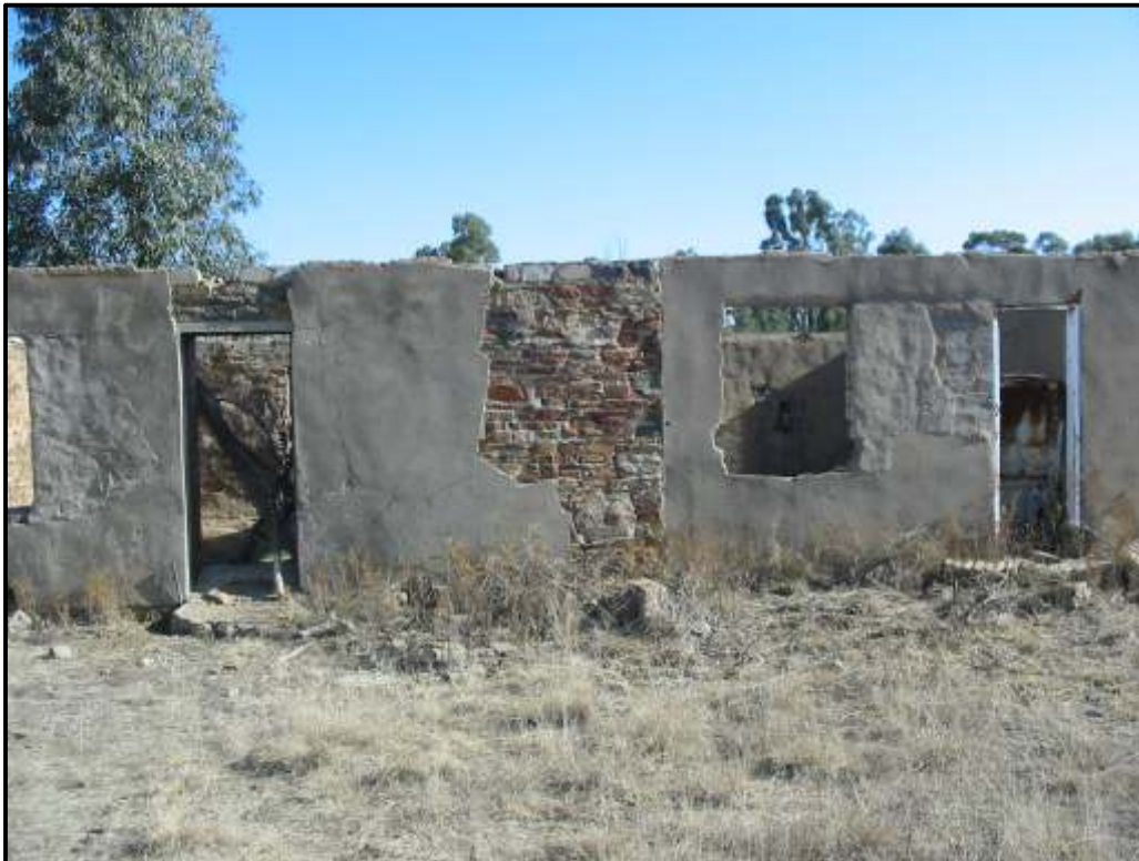
Figure 4: Rectangular structure of stone and cement
