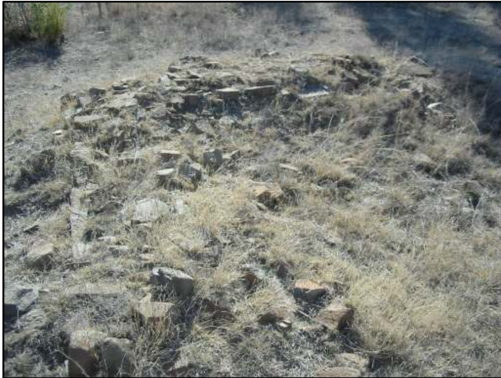
Figure 6: Low stone wall foundations
