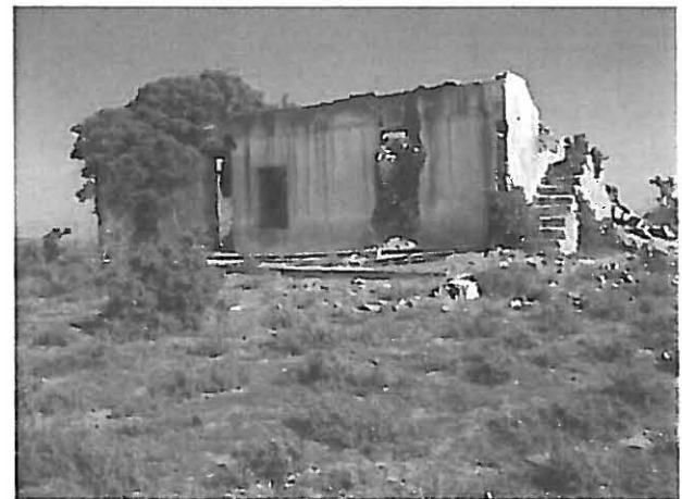
Figure 13. Ruined building on rocky kopje
