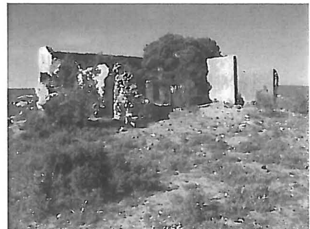
Figure 14. Ruined building on rocky kopje
