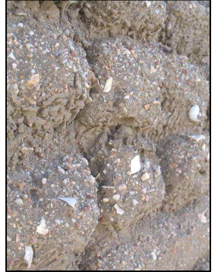
Figure 14: Fragments of shell and flaked stone artefacts embedded in the mud bricks.
