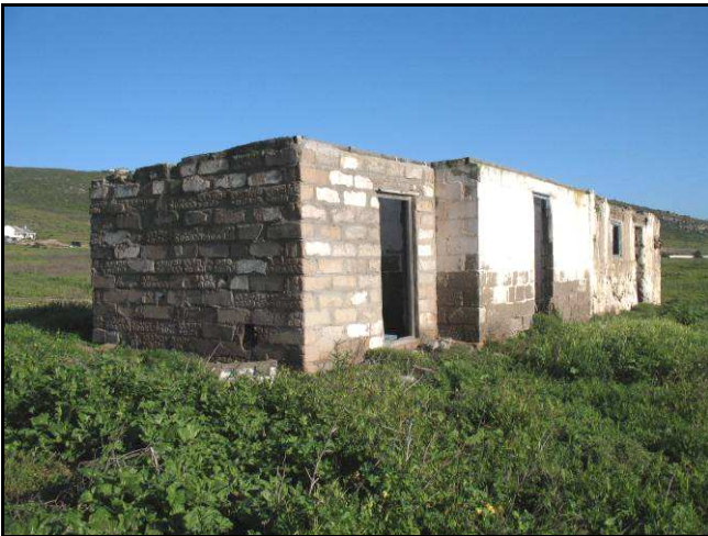
Figure 23: View of the 2 nd addition from the east.
