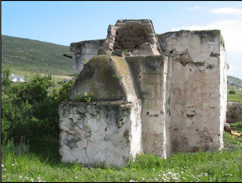
Figure 36: View of the external hearth and chimney stack with attached oven on the southern end of the ruin.
