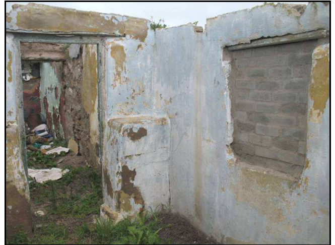
Figure 39: View from the northern addition through the doorways and showing the recently bricked up rear window and the buttress along the original northern wall.
