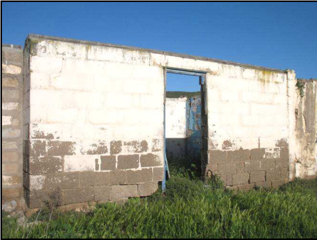
Figure 21: Front view of the 1 st addition.
