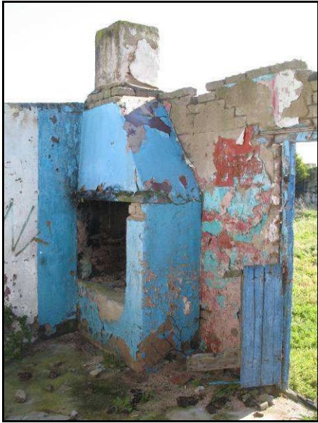
Figure 29: The internal hearth and chimney stack.
