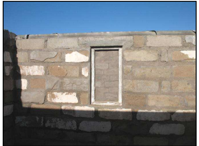
Figure 24: Interior view of the bricked up window.
