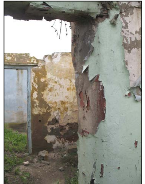
Figure 35: The northern (far) internal door has a wooden frame while the southern one (foreground) has a lintel but no frame.
