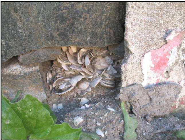
Figure 15: Chunk of palaeobeach deposit included within the wall. It is visible at the bottom in Figure 12.
