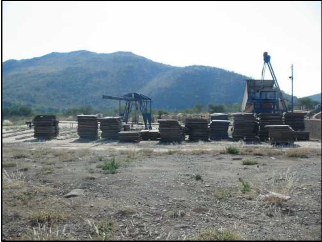
Figure 2: Cement brick factory
