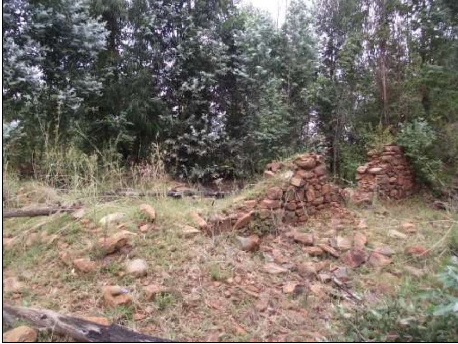
Fig. 23. Site STR 16. Square stone-walled ruin. Probably the remains of farm workers dwelling.
