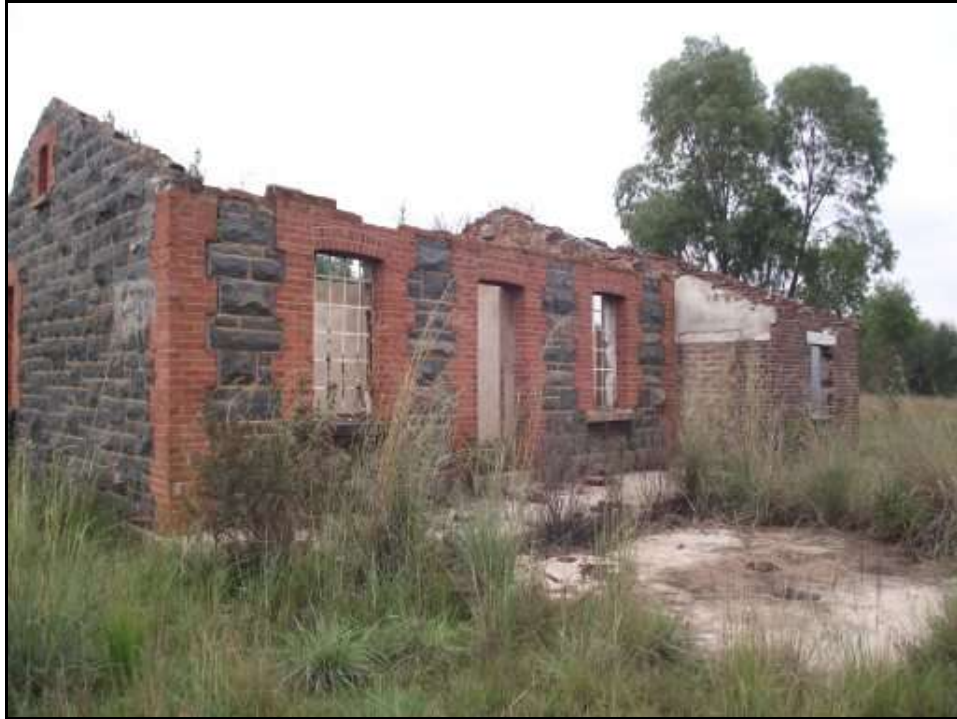
Fig. 1. Site STR 1. Old railway building.
