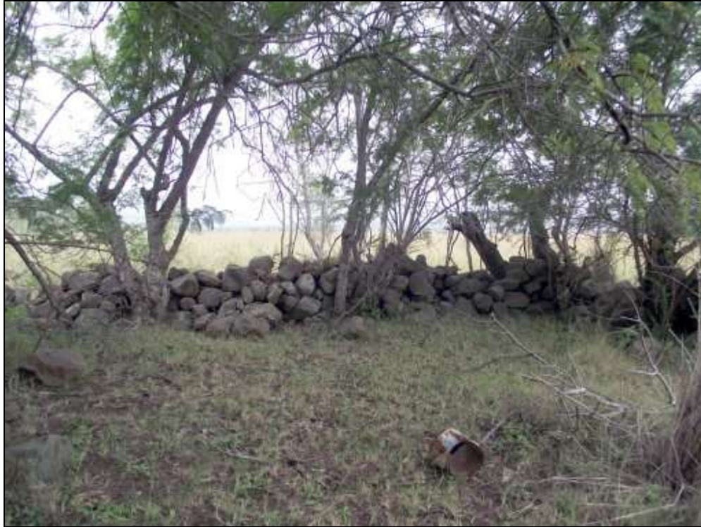
Fig. 19. Site STR 13. Photo taken towards the east.
