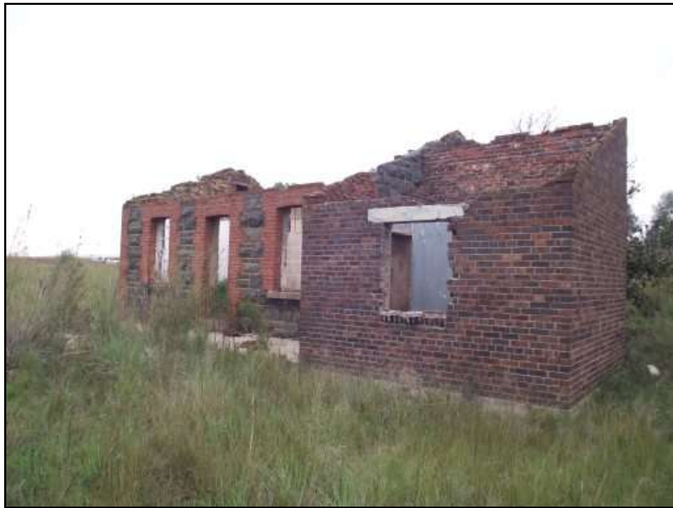
Fig. 2. Site STR 2. Shows additions to original building on the western side.
