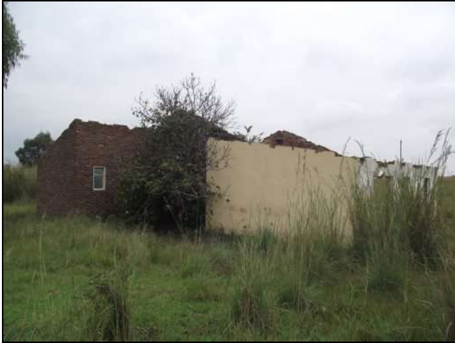
Fig. 3. Site STR 1. Additions to the original building on the eastern side.
