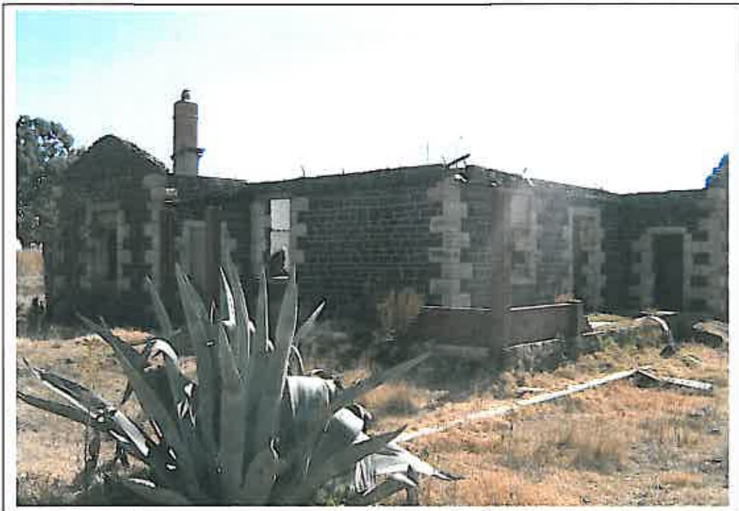
Figure 13 - HH12 was constructed with dolerite and sandstone corner posts and door and window frames (above). This structure is associated with a wagon shed which was constructed with dolerite stone.
