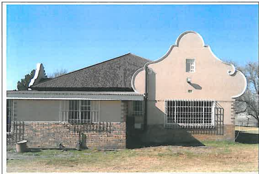
Figure 11- HH07 has been renovated and fitted with new Cape-styled gables (above).
