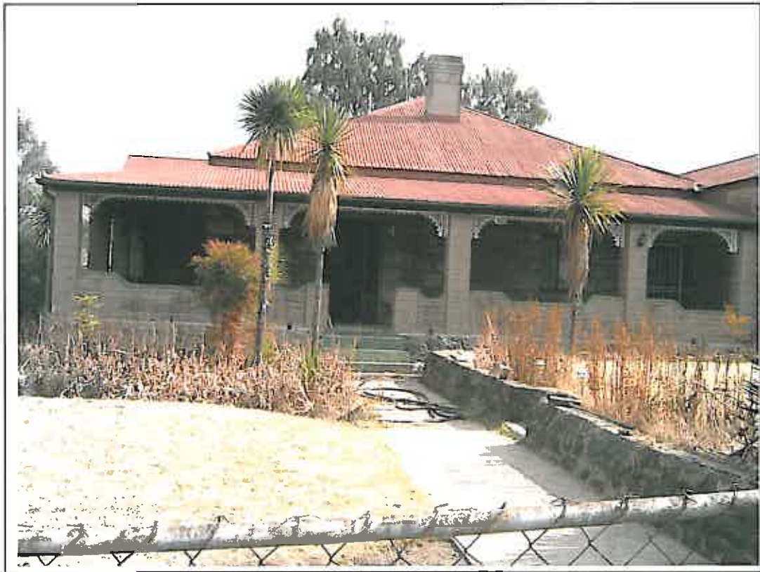
Figure 6- The main residence (FC02.1) constructed with sandstone which is part of FC02. It is associated with a wagon shed (FC02.2) which reveals the same architecture features and building material (above).
