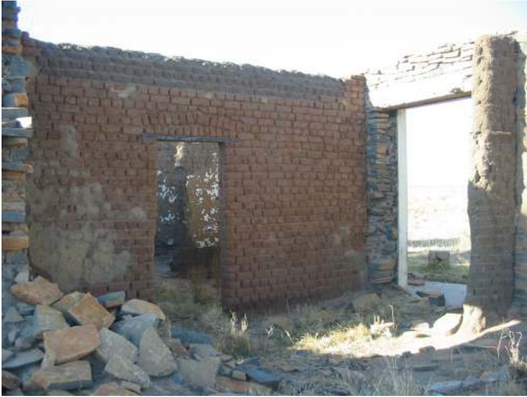
Figure 3: Dilapidated structure. Note the later additions with sun dried bricks
