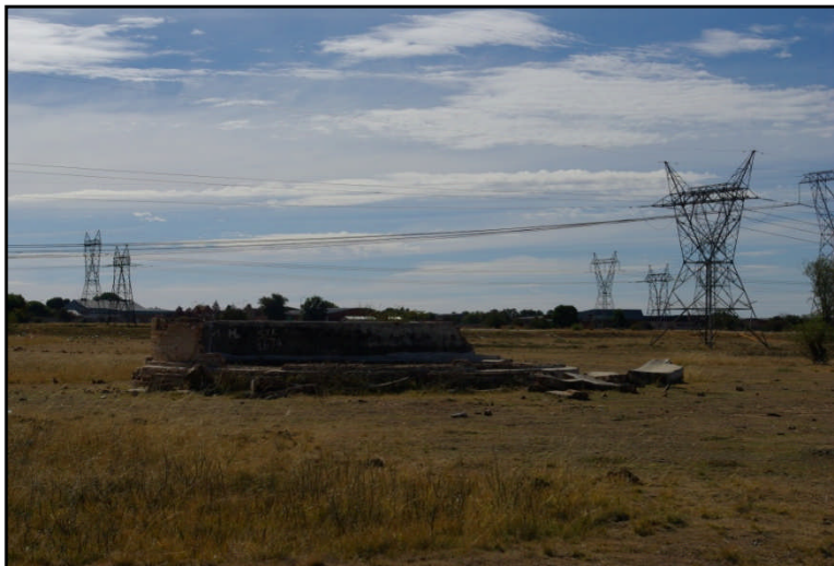
Figure 12: General view of the dam complex
