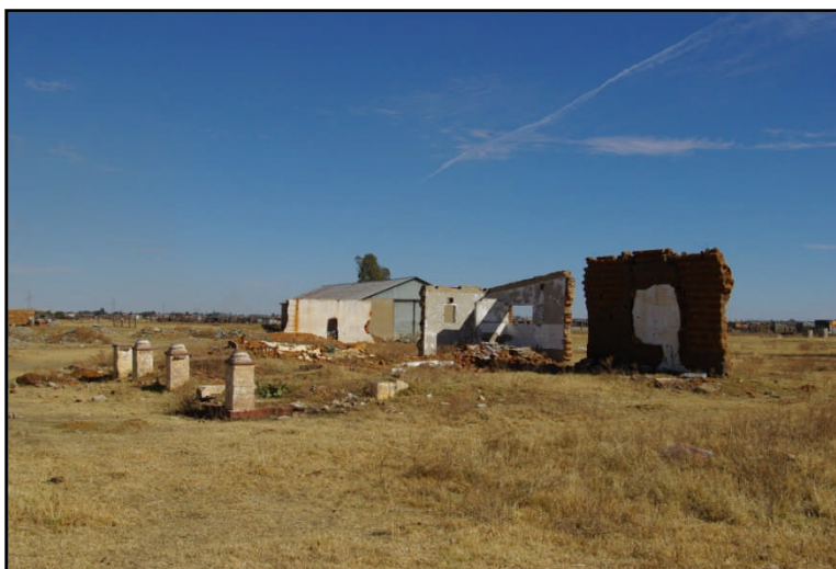
Figure 14: The Site S1 structure 1 remains with the mud brick wall and balustrade and later tiled brick and cement addition clearly identifiable in the foreground and the structure 2 wall in the middleground
