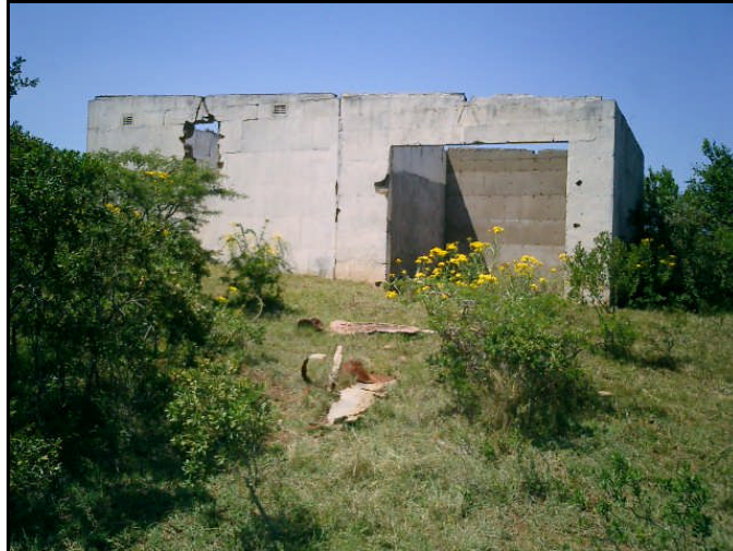
Figure 11: The Site T1 ruined brick and cement structure remains
