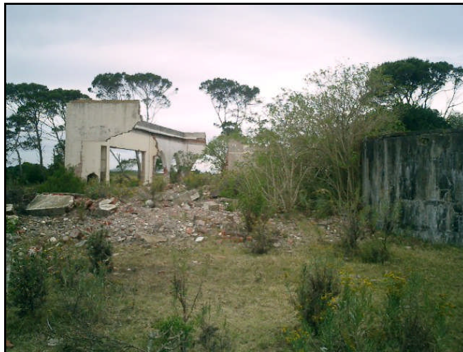
Figure 15: General rear view of Site T2
