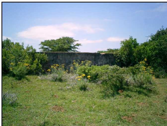
Figure 13: The dam situated in close proximity to Site T1's structure and foundation remains
