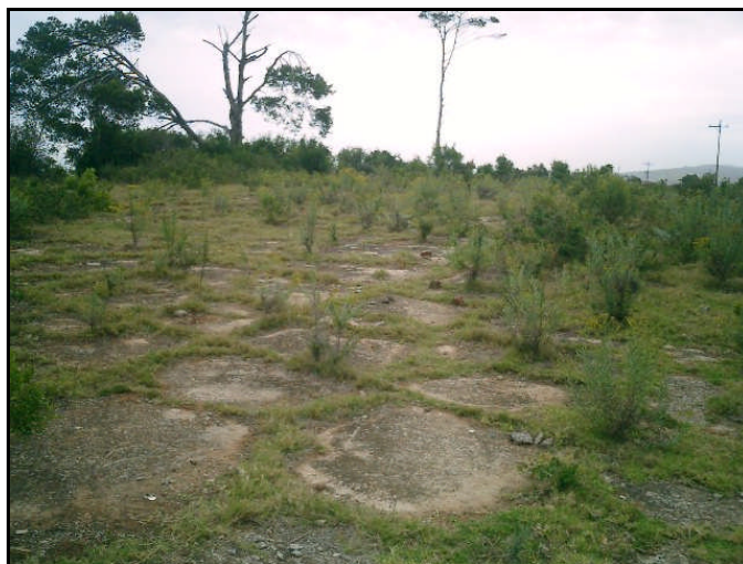
Figure 16: Cement foundation remains located at the back of the Site T2 farmhouse
