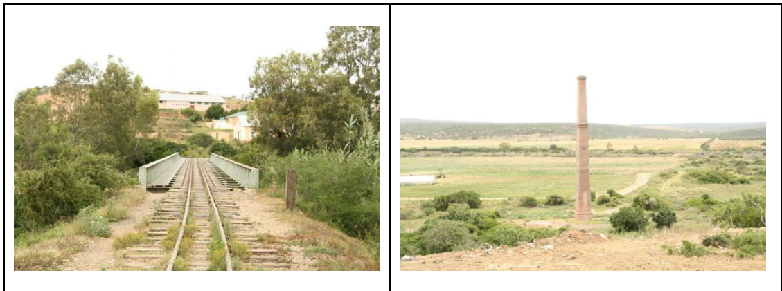
Fig. 12. The narrow gauge railway line across a steel bridge at Hankey and an old brick chimney.
