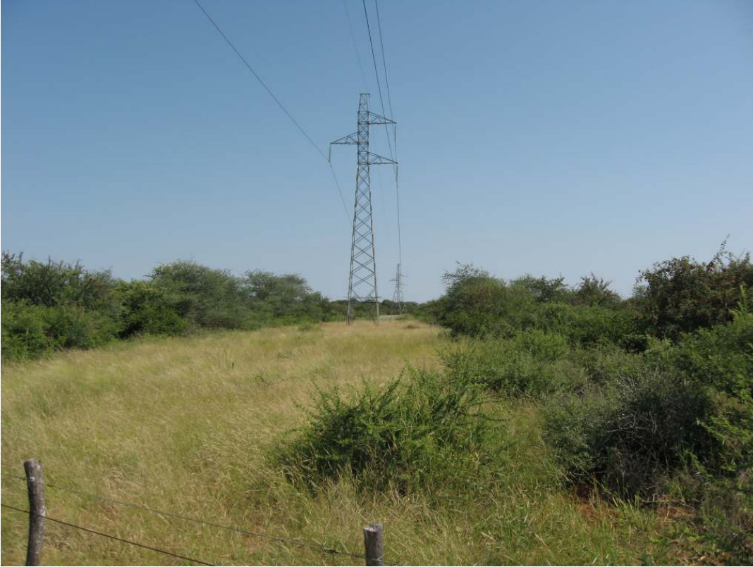
Photo 3: View of the existing power lines across the site.
