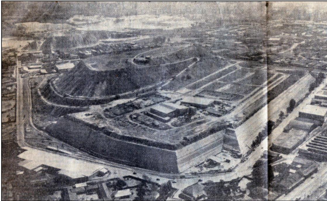
Figure 8 An aerial view of the Top Star Dump in the background, with the tailings dam in front. The photograph appeared in a Rand Daily Mail article of 29 August 1951. The factories that were built on the tailings dam during the 1940s can be seen in the foreground. Note the winding road and single building on the mine dump in the background. The features shown on this photograph correlates with those on the 2628AA topographical sheet for 1956.
