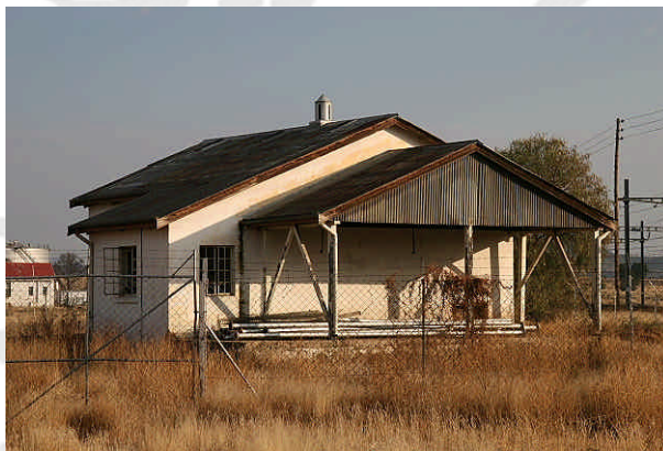
Figure 49: Historic railway shed (old South African Railways – SAR)
