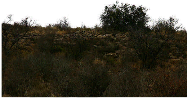
Figure 41: Detail of stone retaining wall at 016.1 Borrow pit
