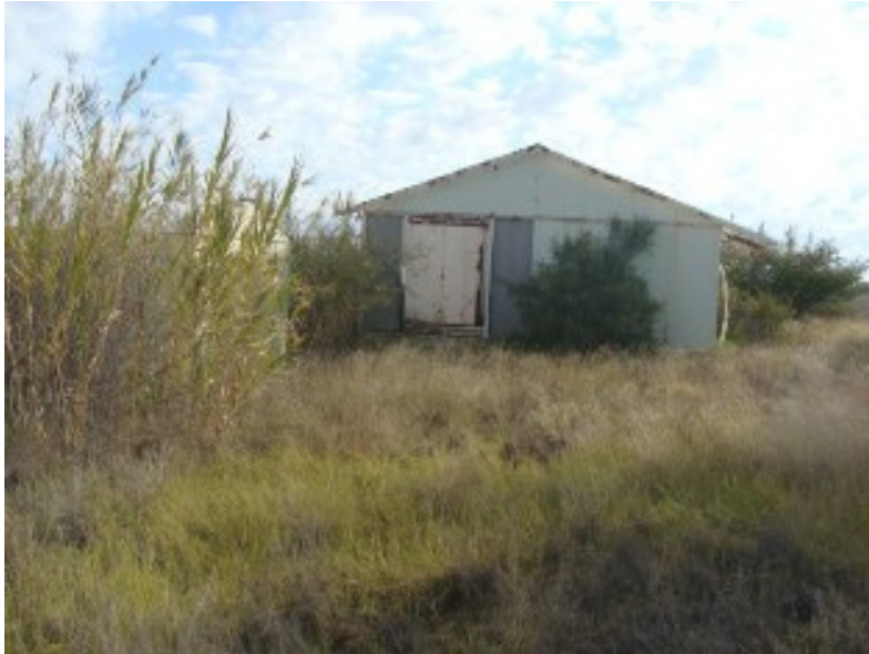
Figure 13: Prefab structure on Site 3
