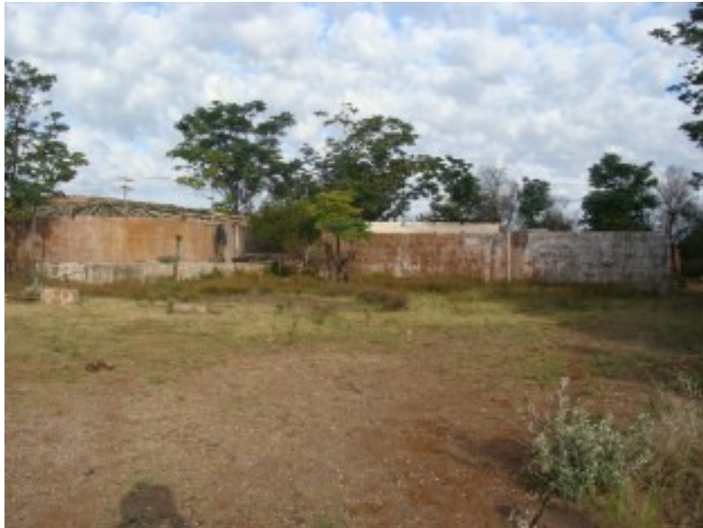
Figure 9: Site 2. The water reservoir/dam is seen on the left side of the picture.
