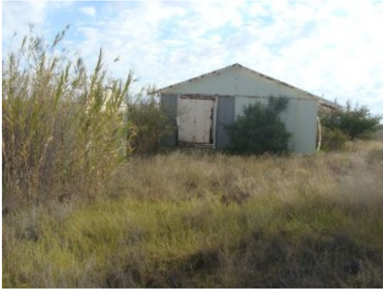
Figure 13: Prefab structure on Site 3
