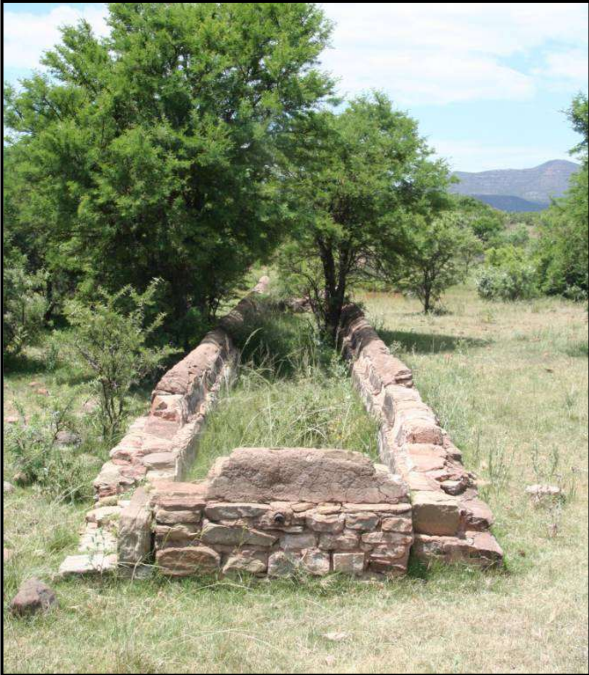
FIG. 7: WATER TROUGH AT TSO02
