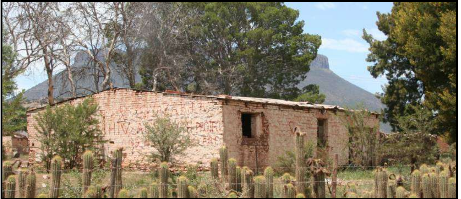
FIG. 9: BUILDINGS AT TS-C1 2
