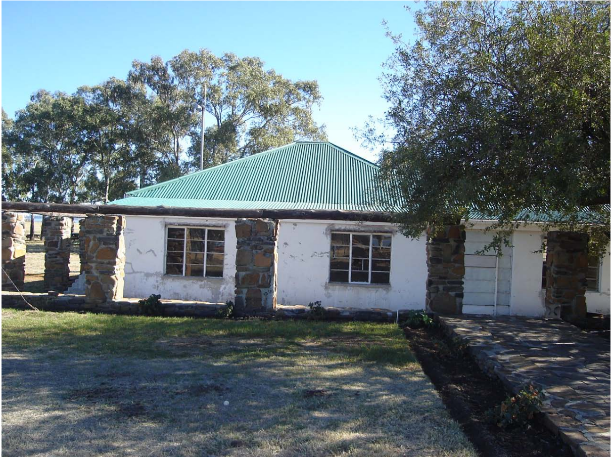
Fig. 3. Old farmhouse on Area 3
