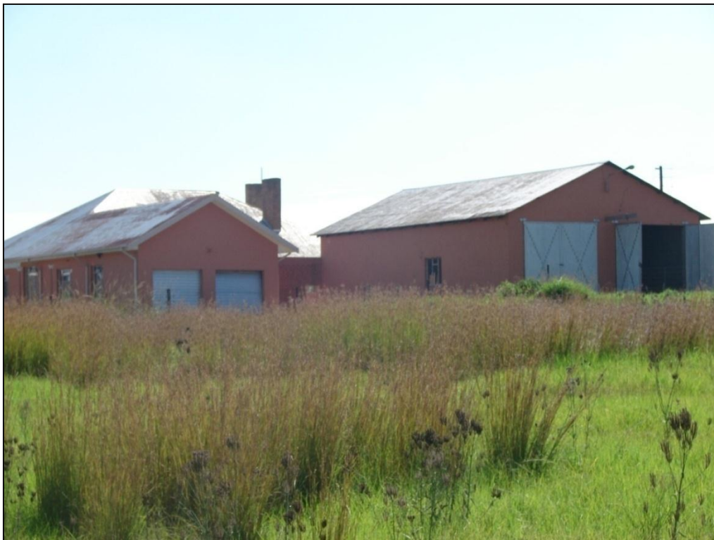
Figure 24 - Shed south of the house in Figure 23. ©Tomose @ PGS.
