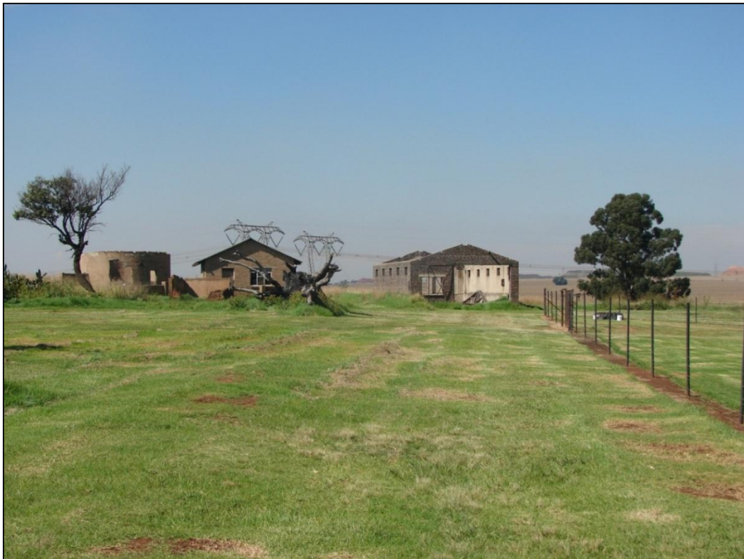
Figure 26 - Dilapidated roundavel, small square structure in front, a modern cottage & dilapidated old shed in fabricated brick- no roof, windows, and door. ©Tomose @ PGS
