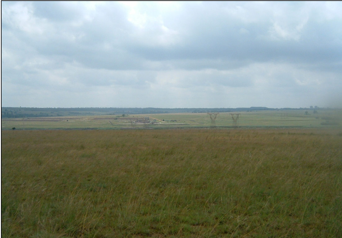
Figure 4- The Kromdraai Collection Pipeline Route runs from the Klipspruit southwards and then eastwards to cross the Brugspruit in order to join the Brugspruit Water Pollution Control Works (far background) above.
