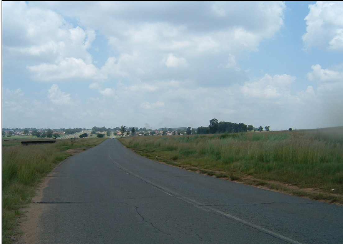
Figure 11- A stretch of the Distribution Pipeline Route runs along the southern shoulder of the R104 which runs parallel with the N4 before joining the KwaGuqa Reservoir further to the west (above).
