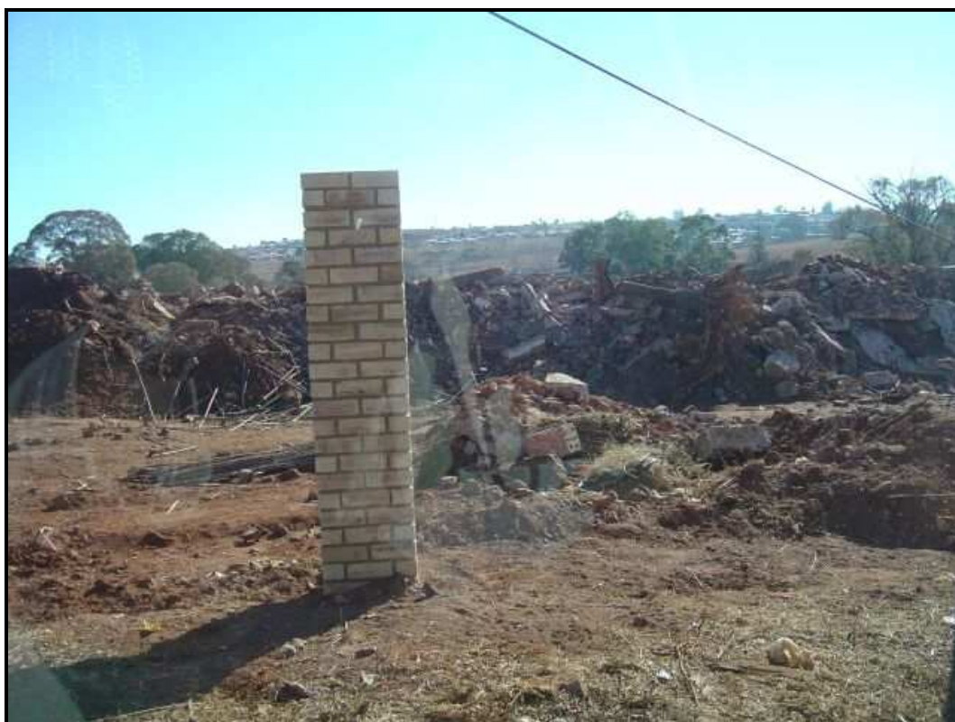
• Figure 3: Remains of houses in south eastern corner of property
