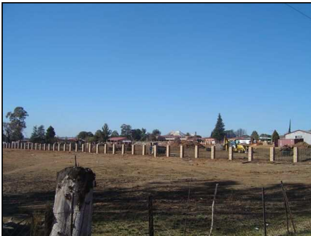
• Figure 2: Construction activities currently on site
