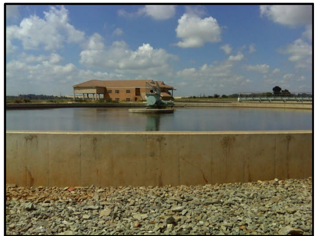
Welgedacht Water Care Works
