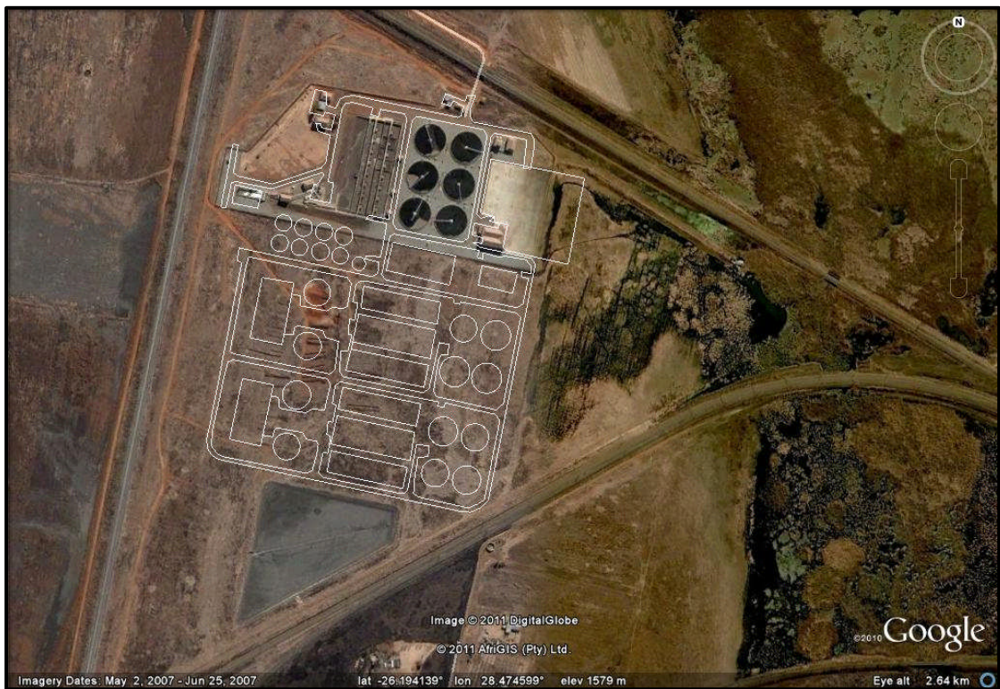
Fig. 6. Proposed extension of the water treatment works. (Photo: Google Earth)
