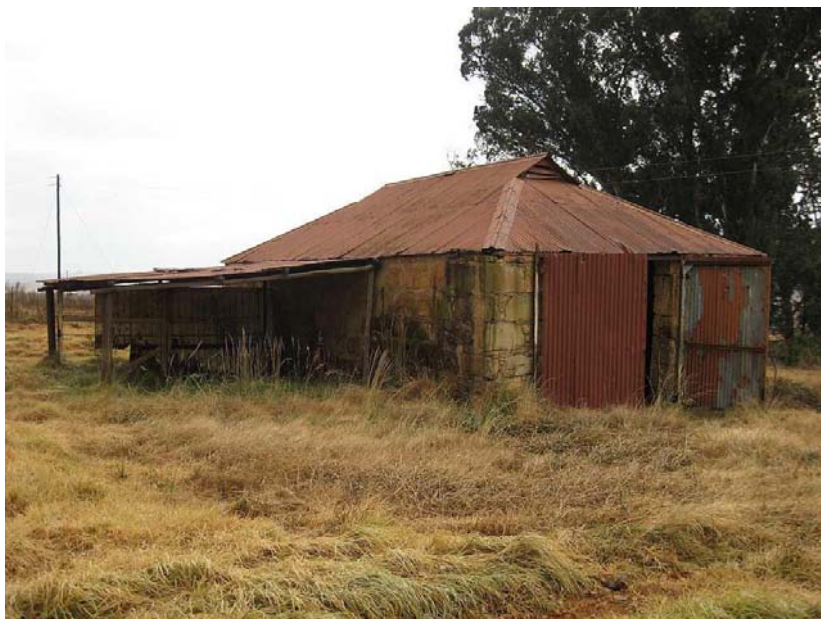
Figure 14. Site WS 4 An old sandstone built shed
