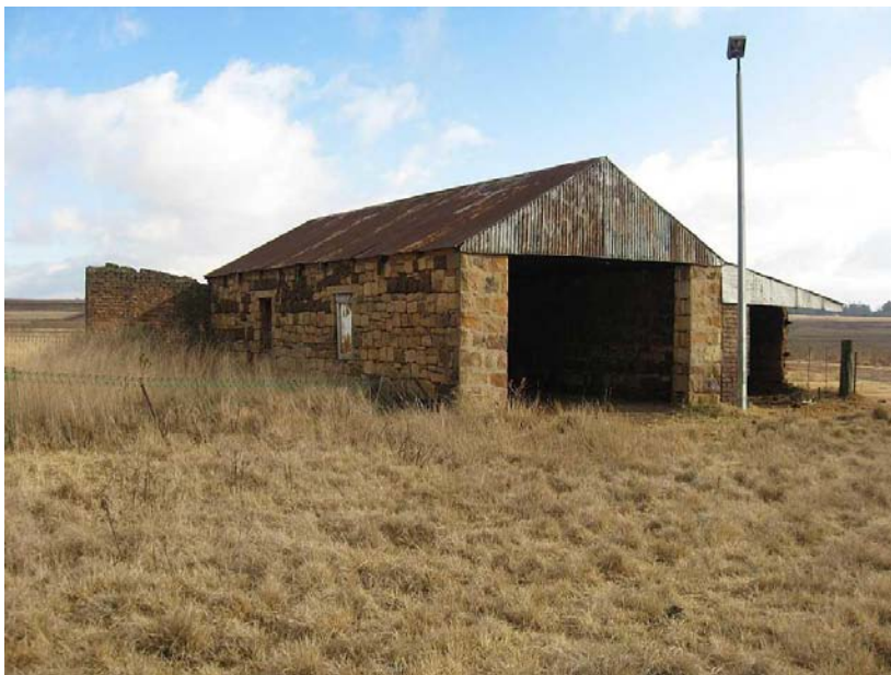
Figure 36. Site WS 11 An old sandstone built shed associated with the old farm house
