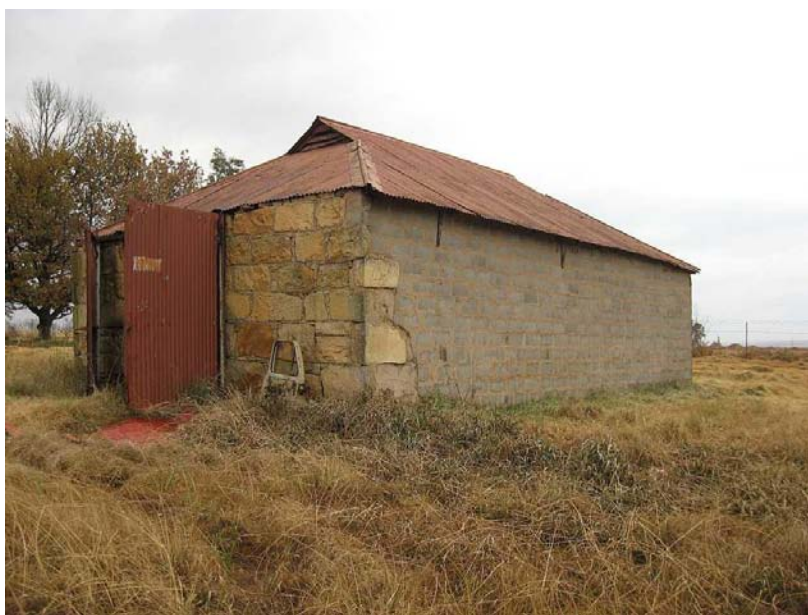
Figure 15. Site WS 4 An old sandstone built shed
