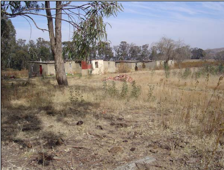
Fig.10 Labourer's houses along the eastern boundary.
