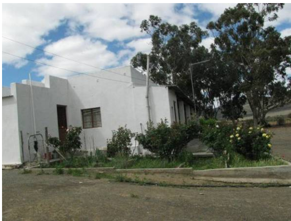
Figure 16 Flat roofed farm house, Haartjieskraal
