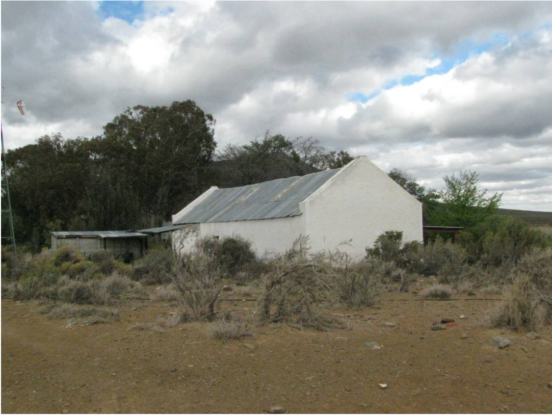
Figure 13 Existing structure, Ekkraal.
