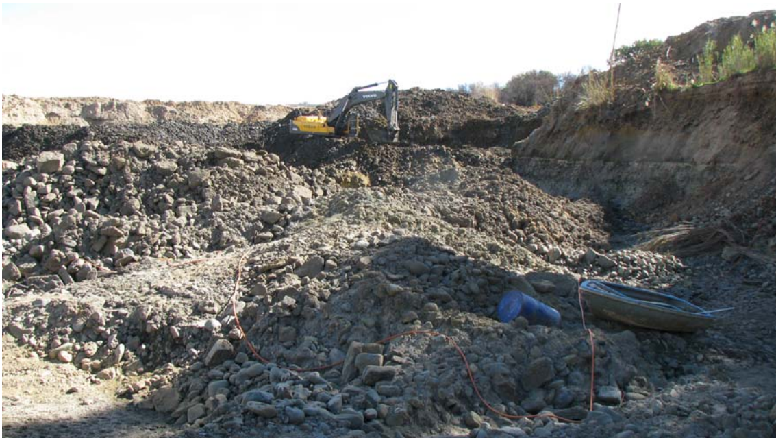
Mining the bed of the river downstream from the island.
