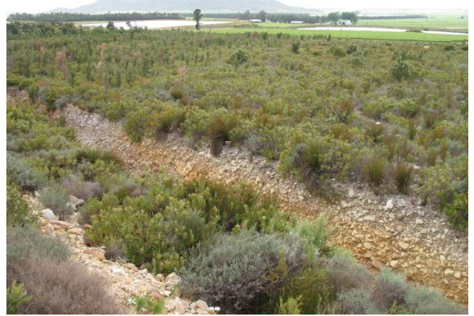
Figure 11. Option C. View facing north. Note the deep excavation trench
