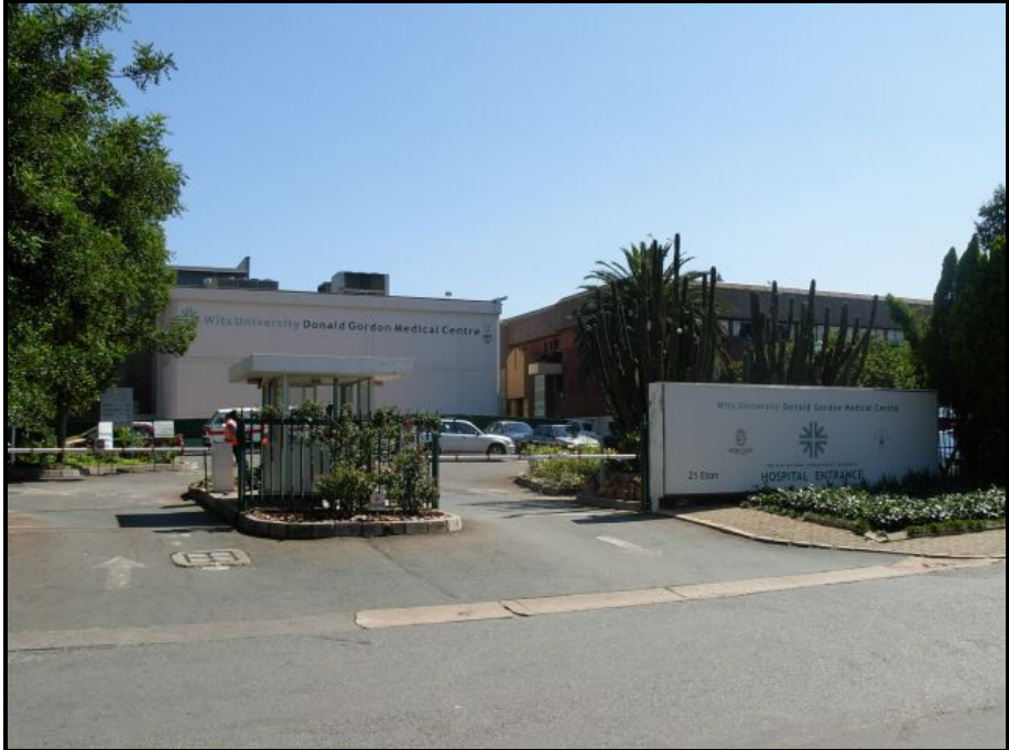
Figure 2: Entrance to WDGMC – to be renovated
