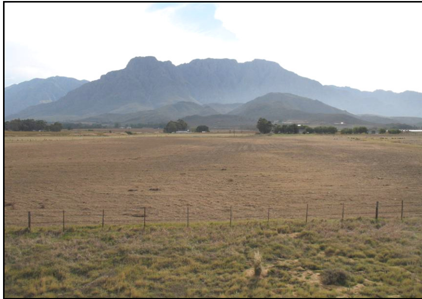
Figure 3: View towards the north over the final northern footprint. A 19 th /early 20 th century farmstead lies in the trees in the right hand background.
