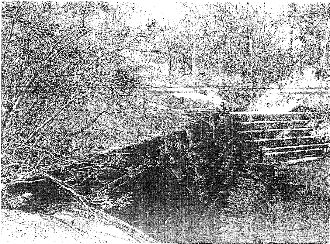
No. 9 The main weir in the Pienaars River from were the water was channelled to the main settlement
