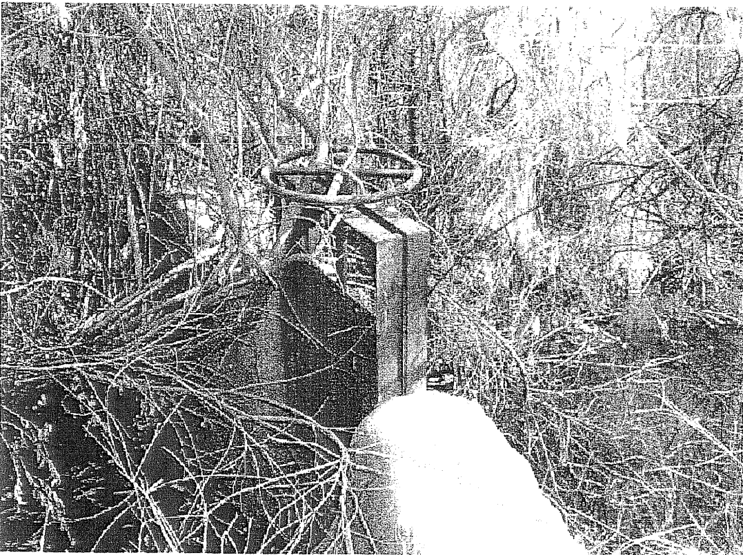
No. 10 Sluice which controlled the water flow in the canal
