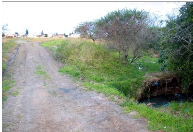
Figure 3: The site where connection bridge is to be constructed, looking south towards the new extension of the King Williamstown cemetery.
