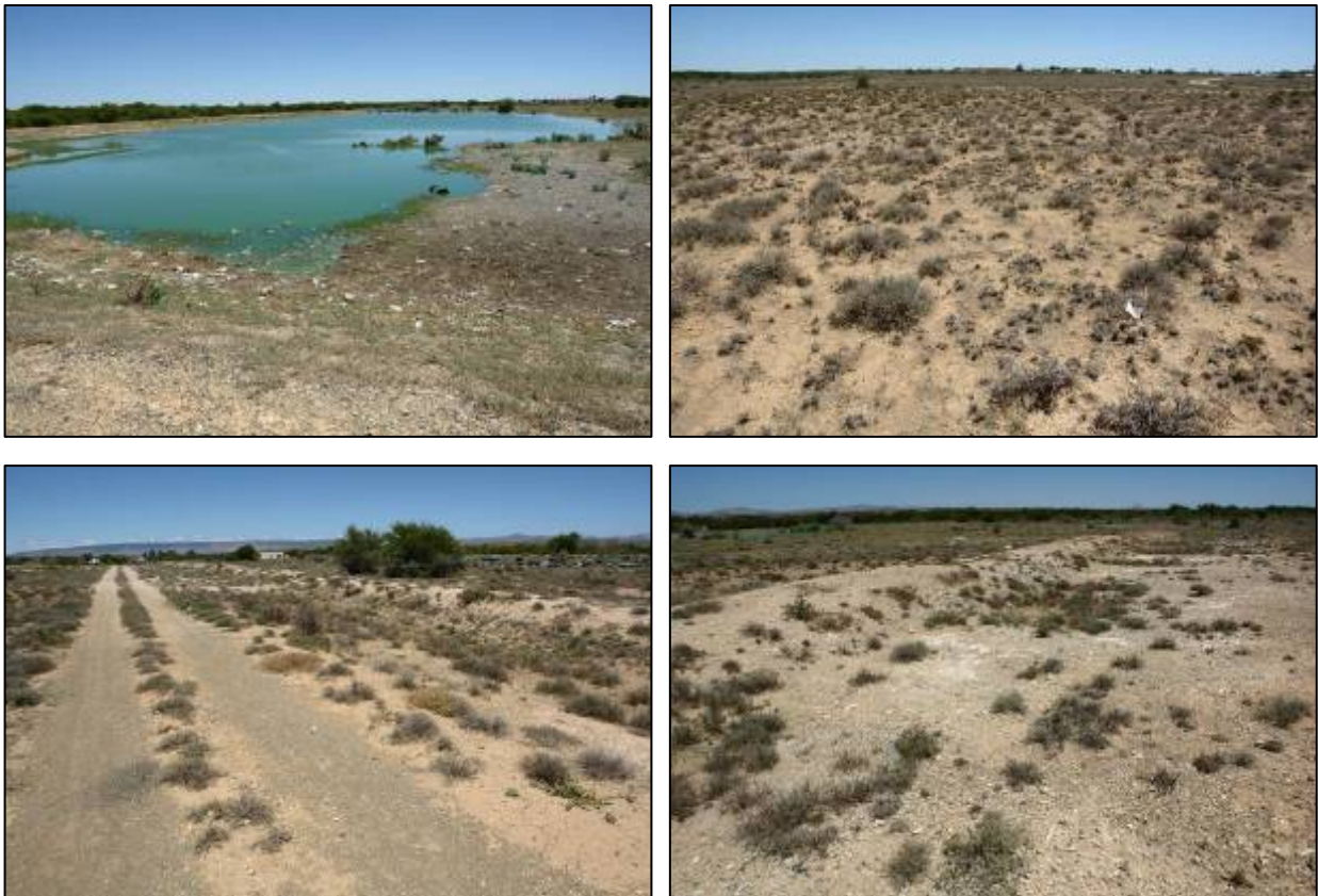
Figs 1-4. Different views of the proposed waste water treatment works to be upgraded in Klipplaai, General views of the waste water treatment works (top left), area between the works and the township (top right) and small scale disturbances adjacent to the works (middle row).
