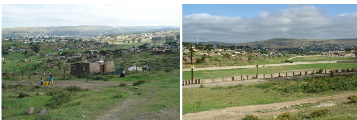
Figs 6-7. A general down hill view of the eastern pipeline route and a view of where the pipeline ends. Note the degree of disturbance to the area.
