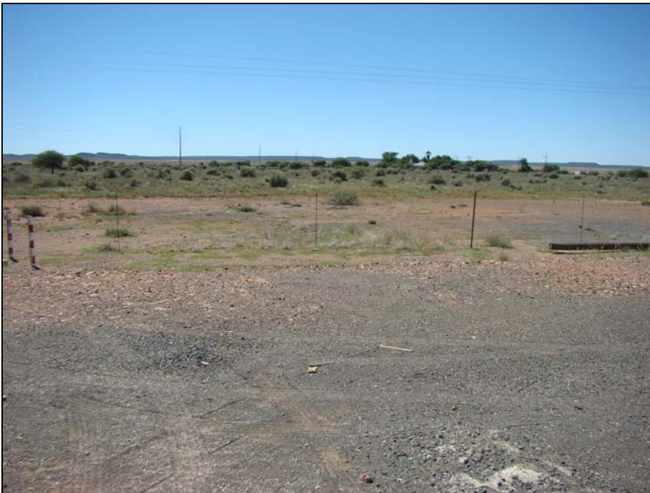
Fig.3 Area around the Osborne Sub-Station at Wicklow 218, Hopetown.
