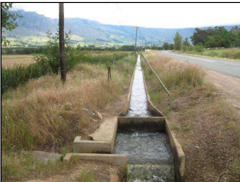
Figure 7. Canal in the road reserve
