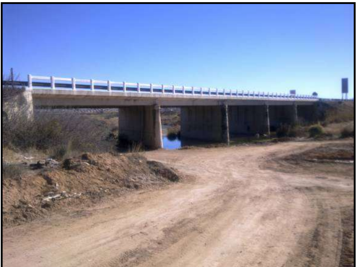
FIG. 13: KLEIN BRAK RIVER BRIDGE
