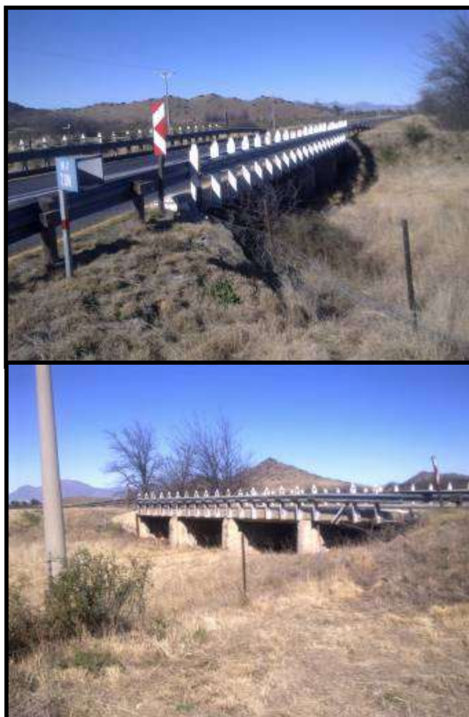
FIG. 16 SELIGMAN BRIDGE: EAST & WEST VIEW
