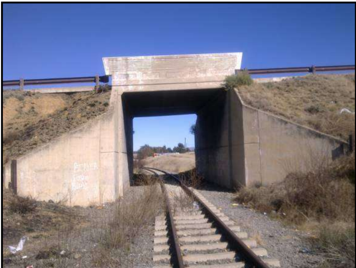
FIG. 12: ROSMEAD ROAD GRADE SEPARATION BRIDGE
