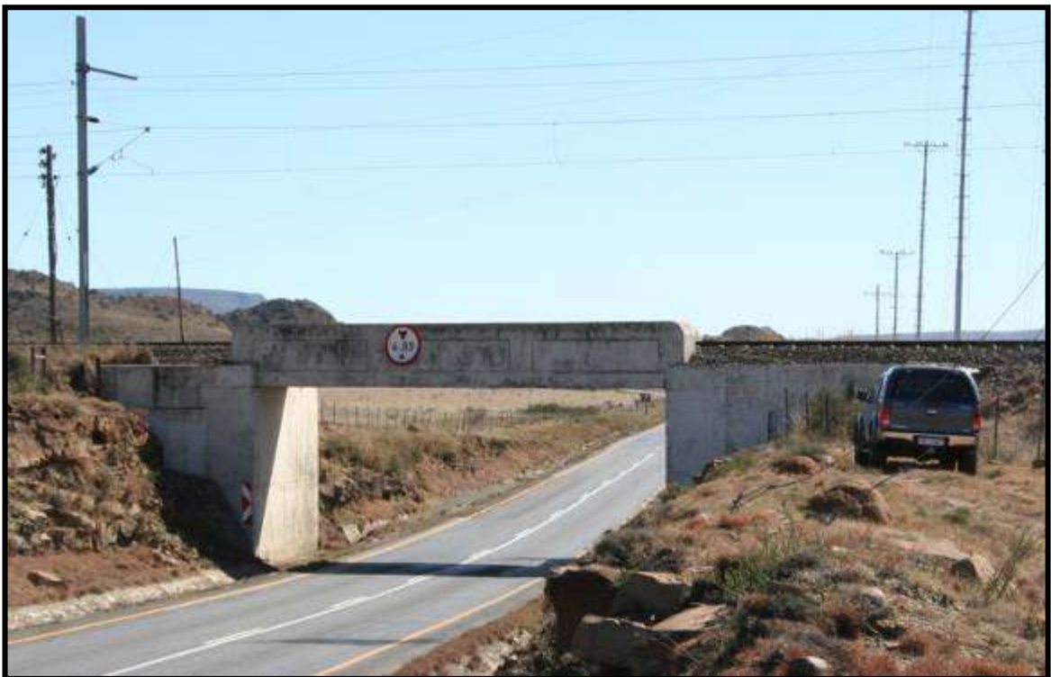
FIG. 17: FLONKERS RAIL BRIDGE
