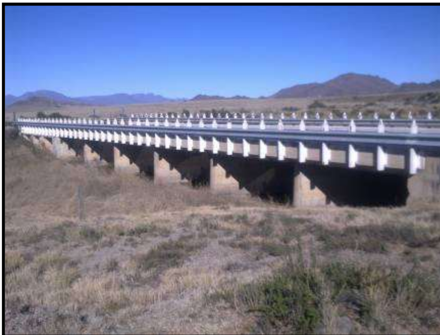
FIG. 15: ELANDSKLOOF STREAM BRIDGE
