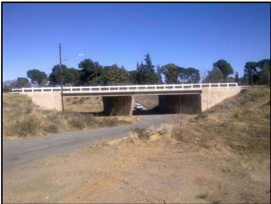
FIG. 14: DROË RIVER BRIDGE
