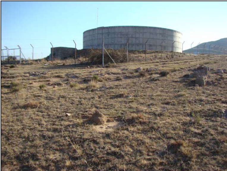
Fig.7 Water reservoir tanks above the proposed landfill site.
